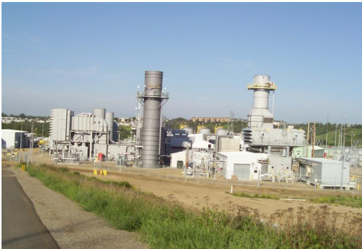
Clover Bar Peaking near Edmonton; GE LM6000, two LMS 100
