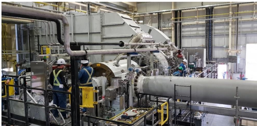
Figure 9: NovaLT16 in TC ENERGY gas pumping station
